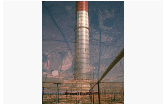
Solar Chimney Manzanares view through the polyester collector roof
