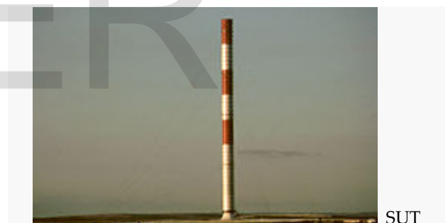
SUT powerplant prototype in Manzanares, Spain, seen from a point 8 km to the South
